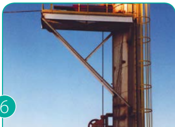
6 Barge System Terminal Flag Fairlead Sheaves
